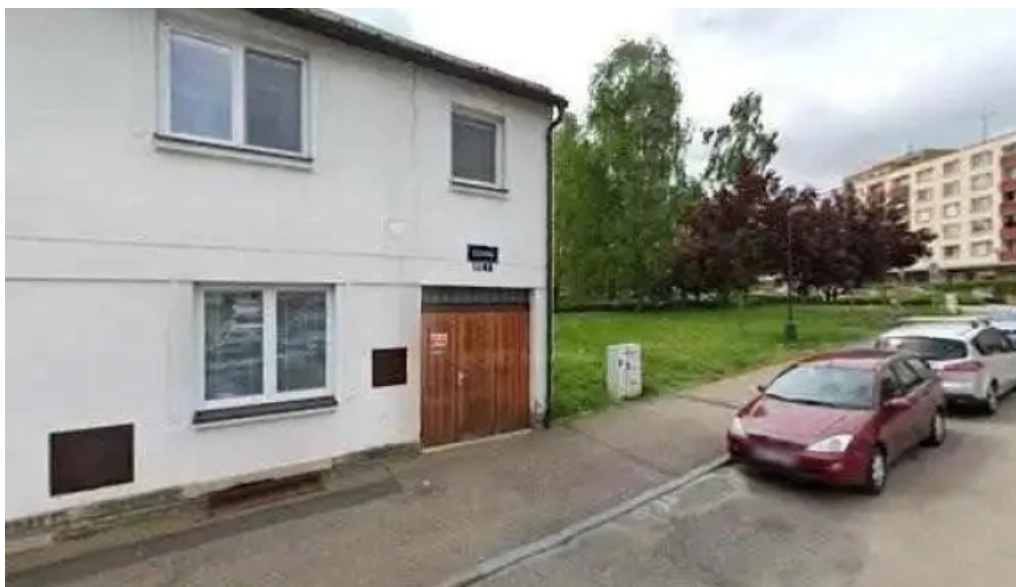
Restaurace na zachytce street view a 360deg
