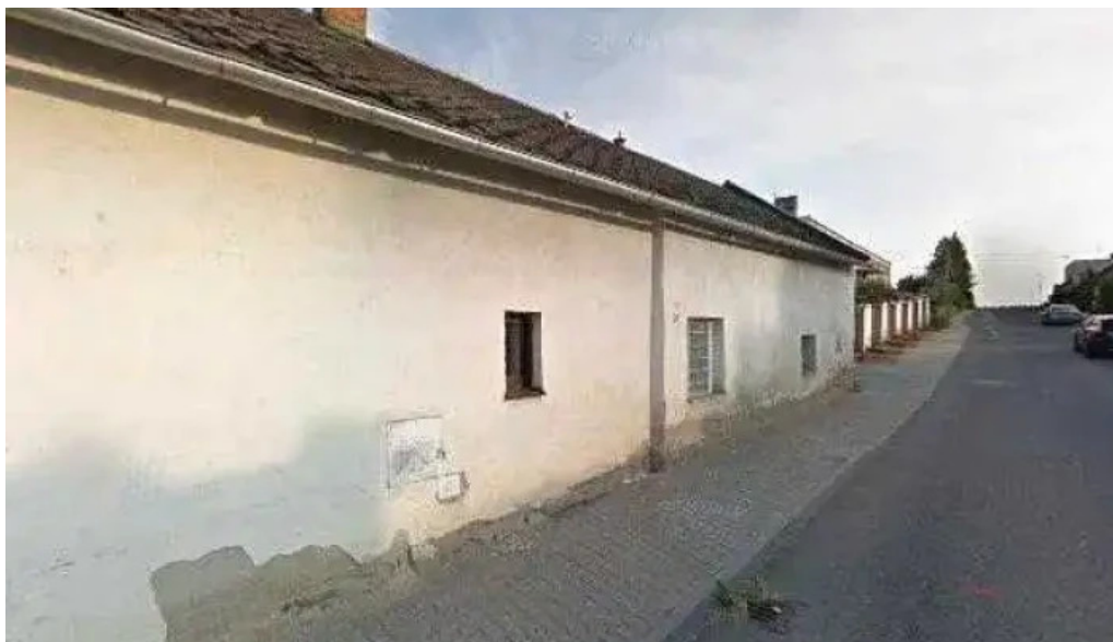
Restaurace na zatacce street view a 360deg
