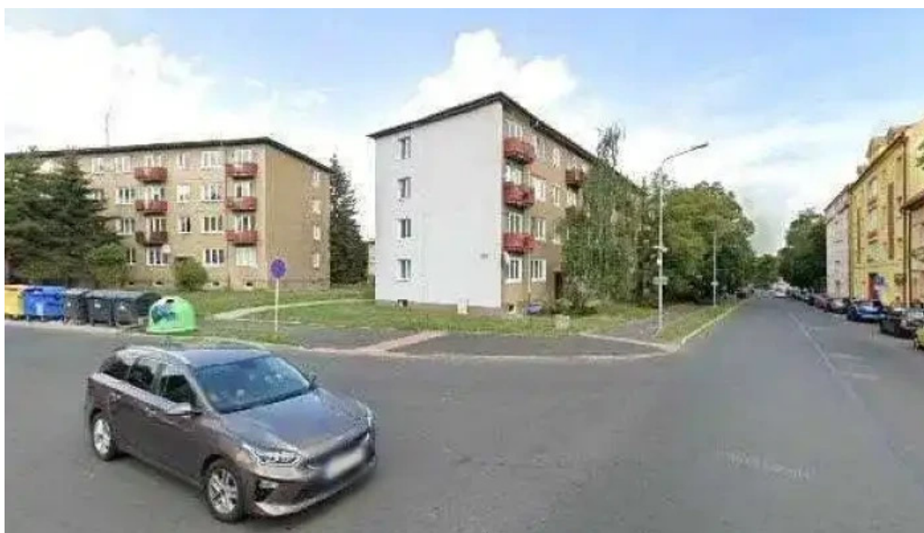
Restaurace barborka street view a 360deg
