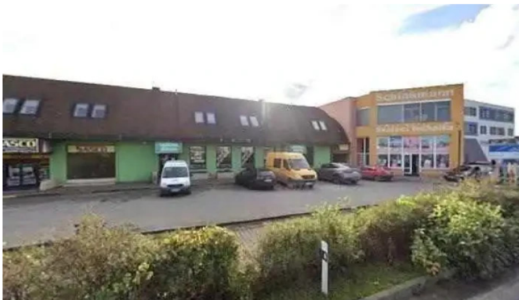
Restaurace abasta street view a 360deg
