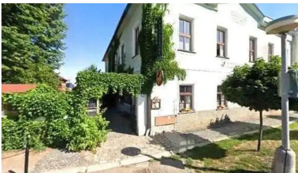
Restaurace a penzion u hajku street view a 360deg
