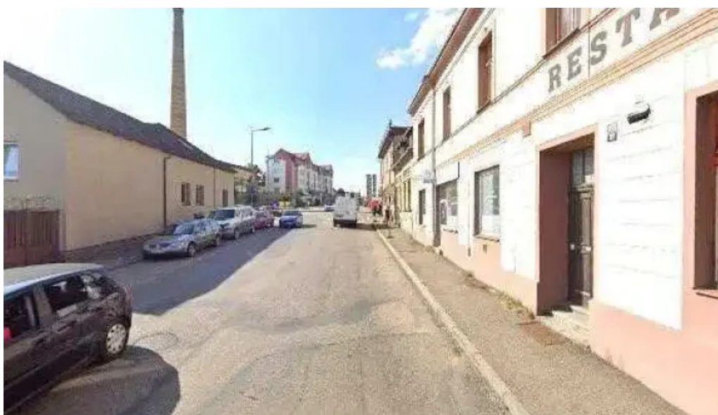
Restaurace na tumovce street view a 360deg
