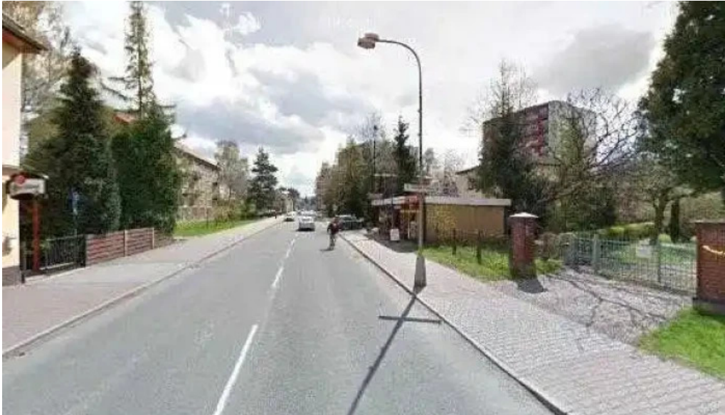
Iphone servis industries street view a 360
