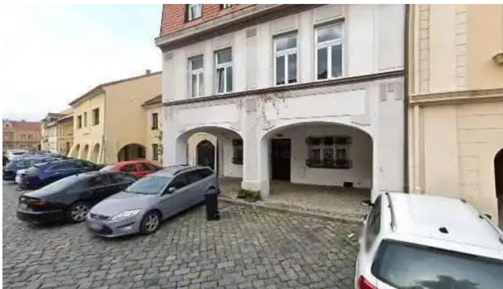
Hotel u cisare street view a 360deg
