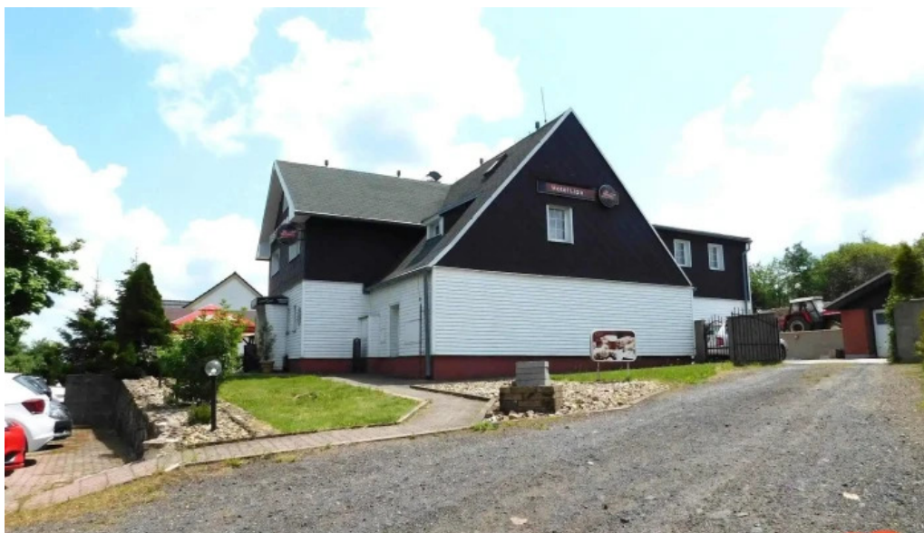
Hotel linde hotel a restaurace lipa cinovec exterier
